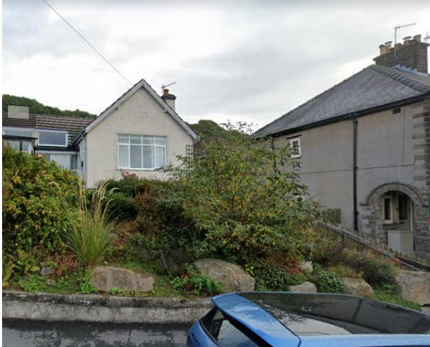
Site prior to works.
